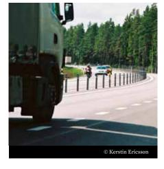
• A new and widely discussed innovation is the **2+1 lane highway with a median barrier**, a road type developed in Sweden.
