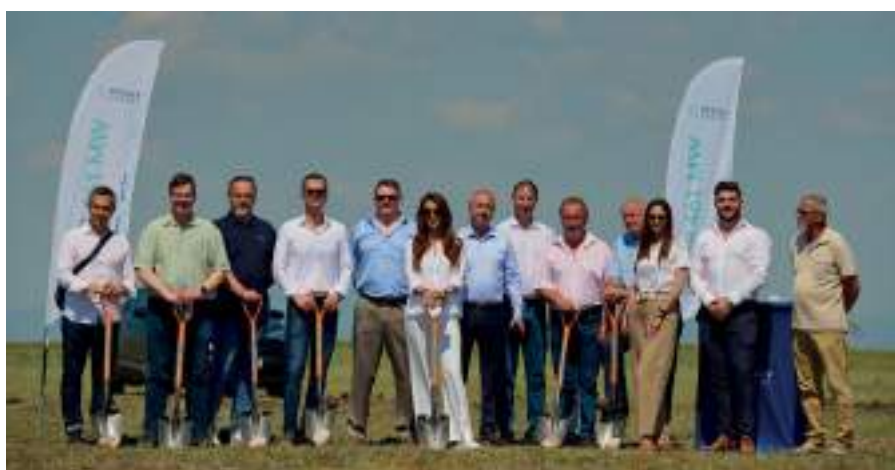
Rezolv Energy and project partners break ground at the VIFOR wind farm in Buzău County, Romania
